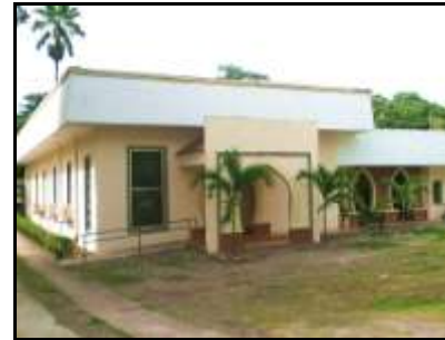
SOCIAL/FUNCTION HALL BLDG.
