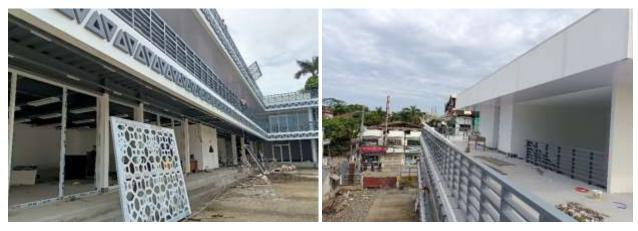
The Construction of the Two (2) Storey with Roof deck SPDA Veterans Office Building was commenced in the **First Quarter of CY 2022**. It started with the demolition and clearing of the project site old structures and other unnecessary objects. Excavation of protection/sheet piles along the properties affected during foundation excavations, building foundations and pedestals, and so with the retaining walls of the ground floor level were also completed.
