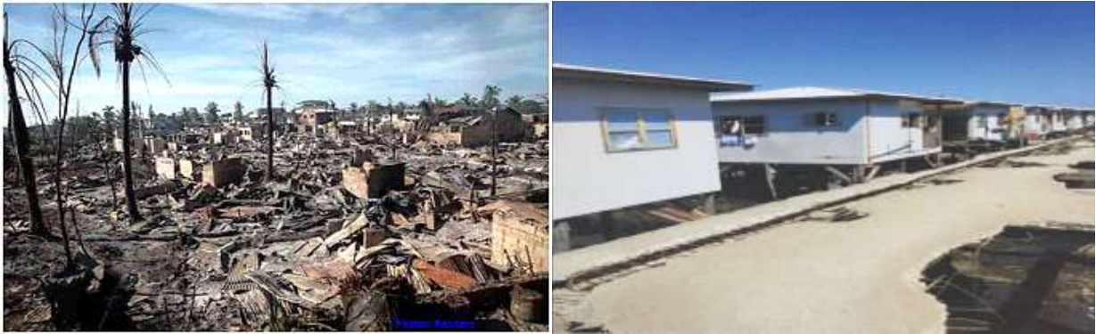
Before and after pictures of the SPDA Rio Hondo Property, Zamboanga
